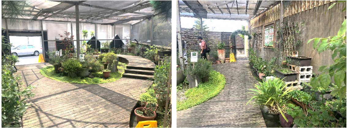
圖三、園區原設置噴灌系統，長期濕度高，造成木棧道潮濕形成青苔與濕滑，牆面也變成深灰色。 Fig. 3. The humidity of the herb garden was high, the wooden walkway was damp, mossy and slippery.
